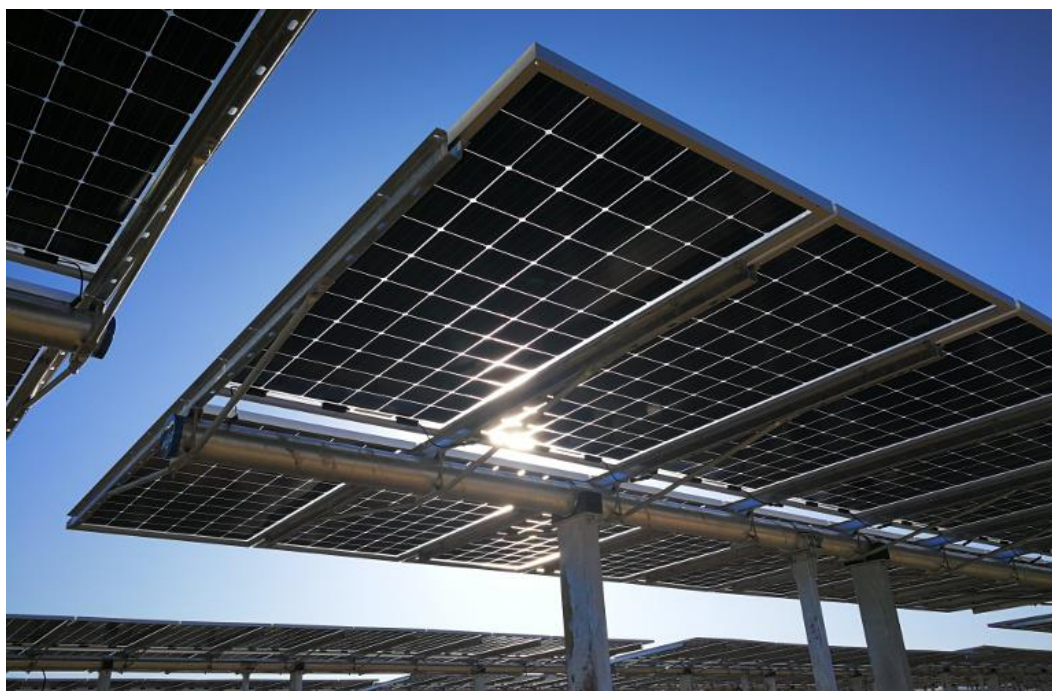
Figure 11: Single access tracking solar farm with bi-facial panels 7
